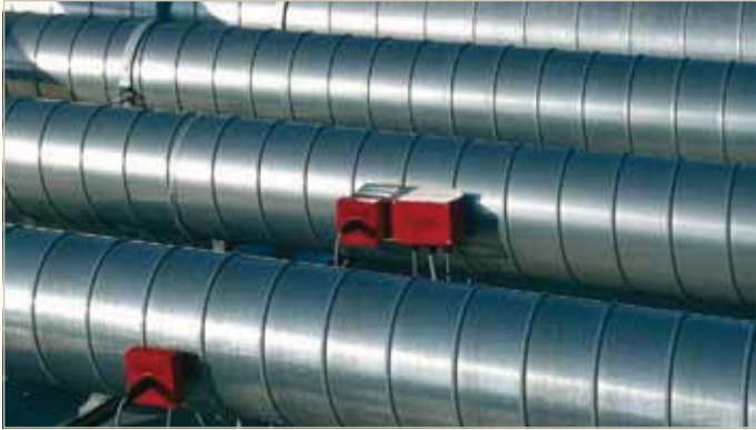
Extraction system with spark detectors
