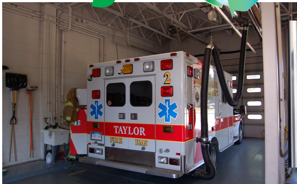
The magnet on the hose attaches to an anchor plate on the vehicle.
